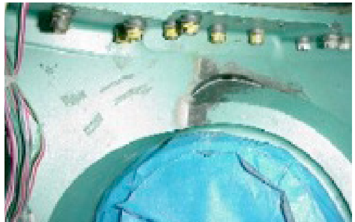
The result: the repair is performed flawlessly.
